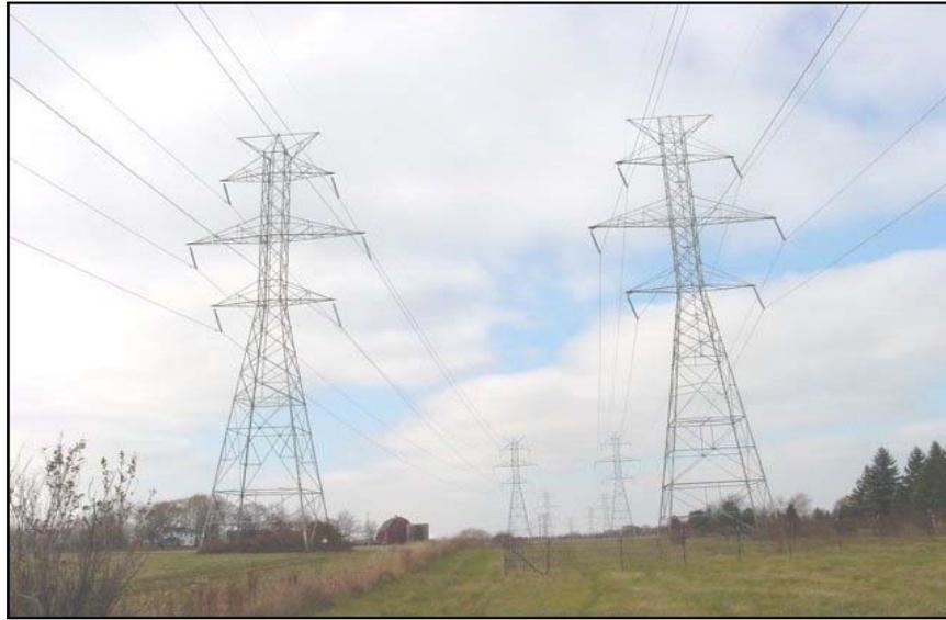
**Figure 3 Close-up of a Double-Circuit Transmission Structure**
